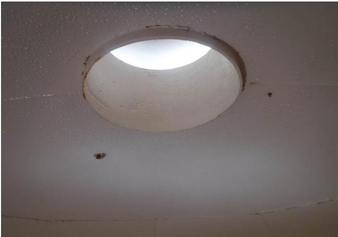
Interior Coating Roof
