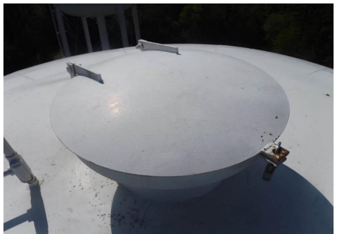
Exterior Coating Roof
