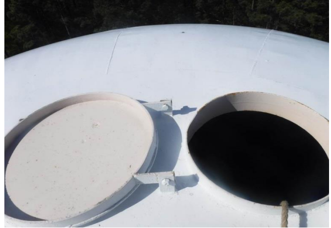
Wet Interior Access Hatch Open
