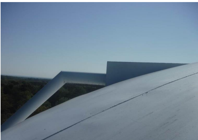
Exterior Coating Roof
