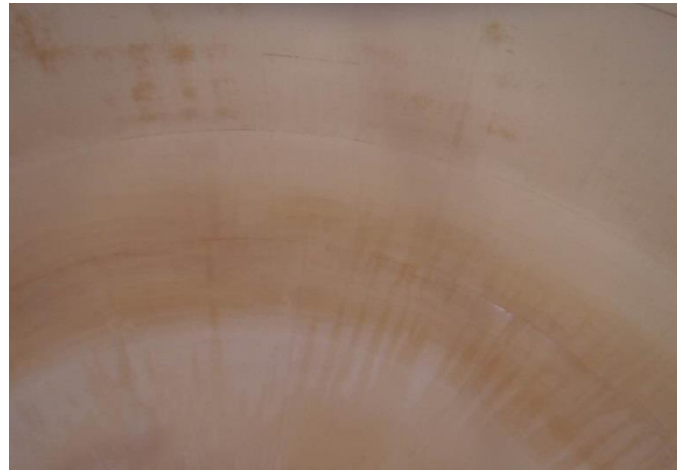
Interior Coating Sidewall
