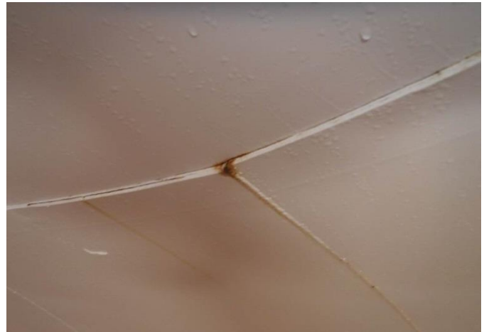
Interior Coating Roof
