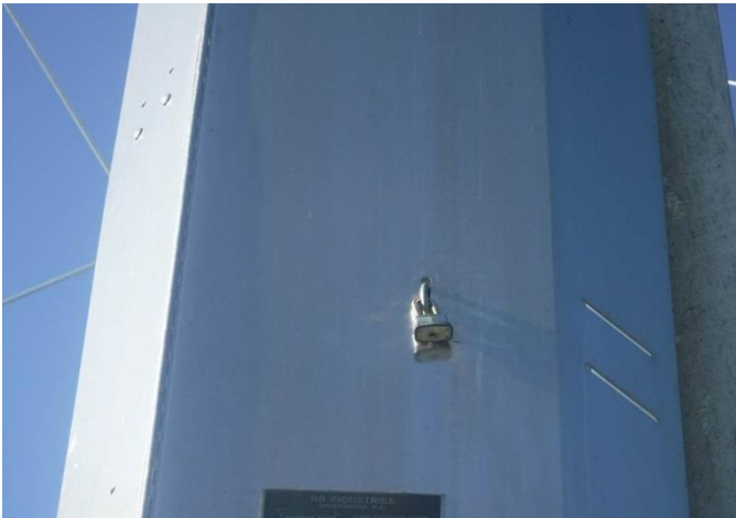
Ladder Guard Locked
