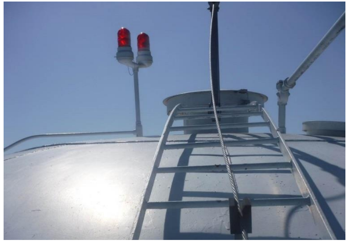
Exterior Coating Roof
