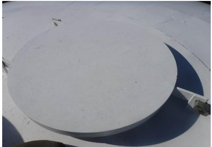
Access Hatch Locked
