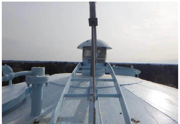
Exterior Coating Roof
