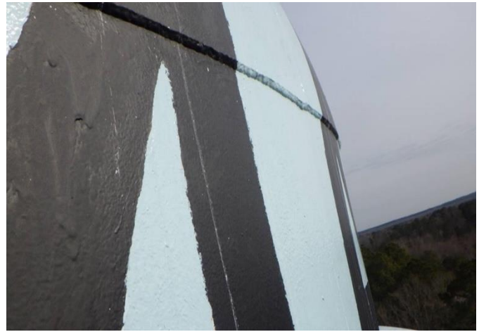
Exterior Coating Sidewall
