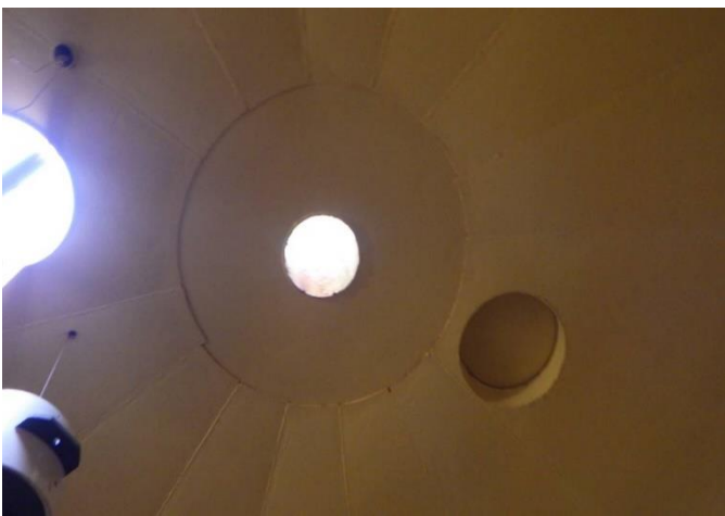
Interior Roof Structure
