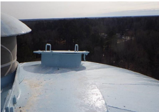
Exterior Coating Roof
