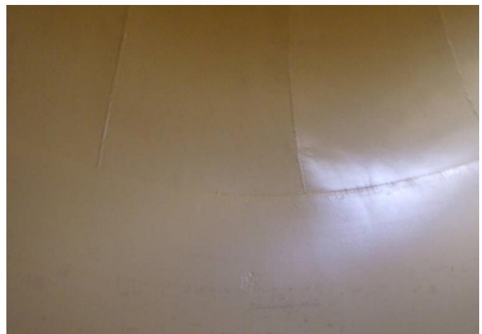
Interior Coating Roof and Sidewall
