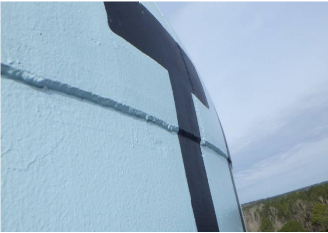
Exterior Coating Sidewall
