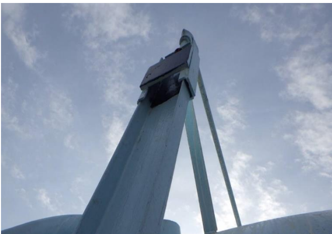
Float system Repaired
