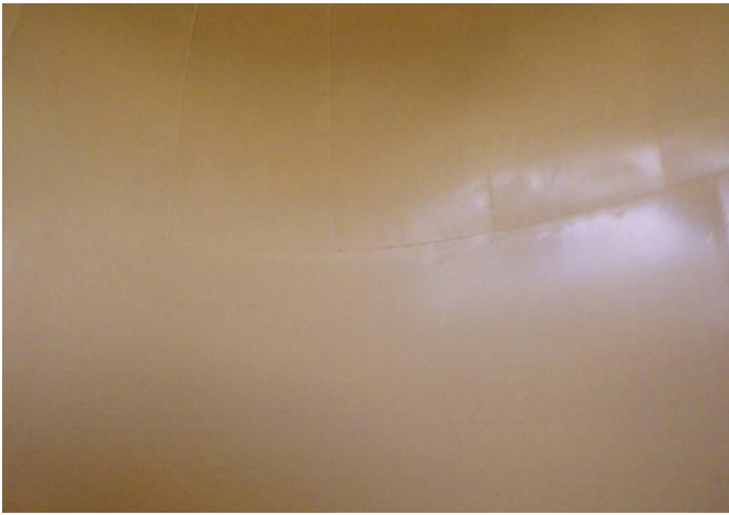
Interior Coating Roof and Sidewall
