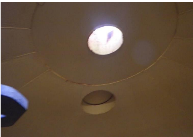
Interior Coating Roof
