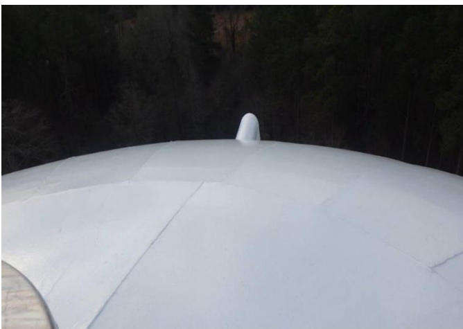
Exterior Coating Roof
