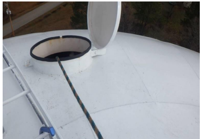
Wet Interior Access Hatch Open
