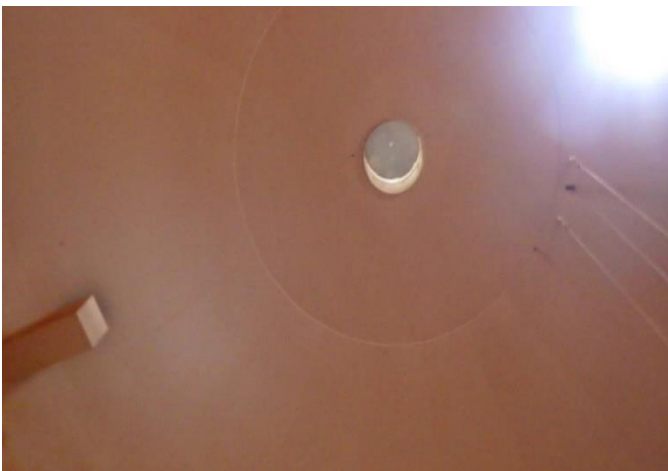
Interior Roof Structure
