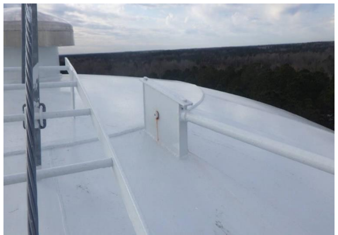
Exterior Coating Roof
