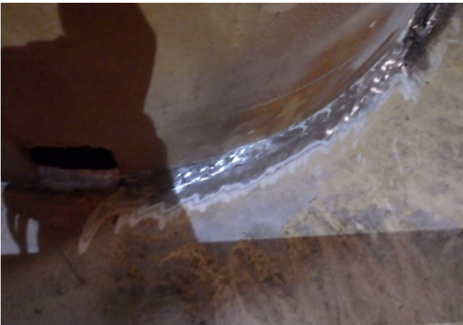
Bowl/Riser Connection Repairs Prior Painting
