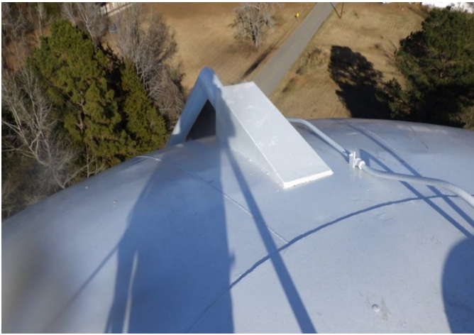
Exterior Coating Roof
