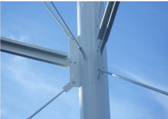
Strut Connections
