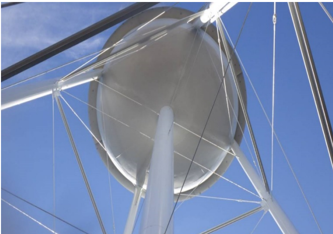
Exterior Coating Under Belly
