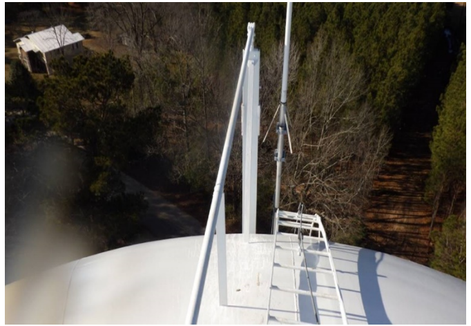
Exterior Coating Roof
