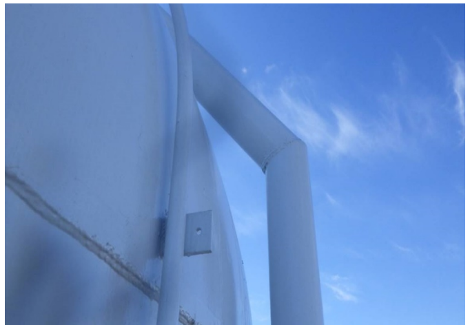
Exterior Coating Sidewall
